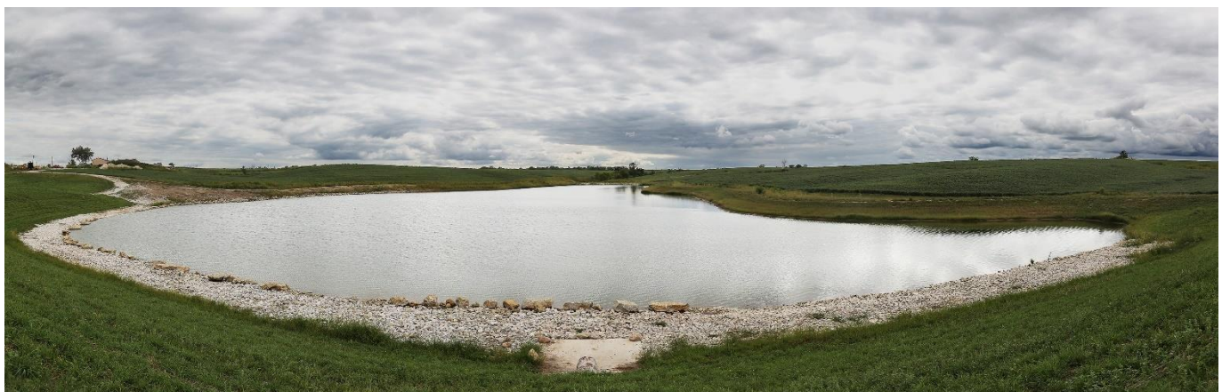
Figure 4. Farm pond constructed in the Soap Creek Watershed designed to capture runoff and reduce flooding.
